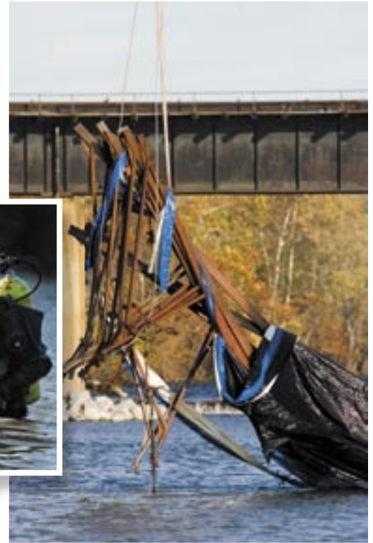
Divers work on removal of the portable dam and sandbags that held it in place.
